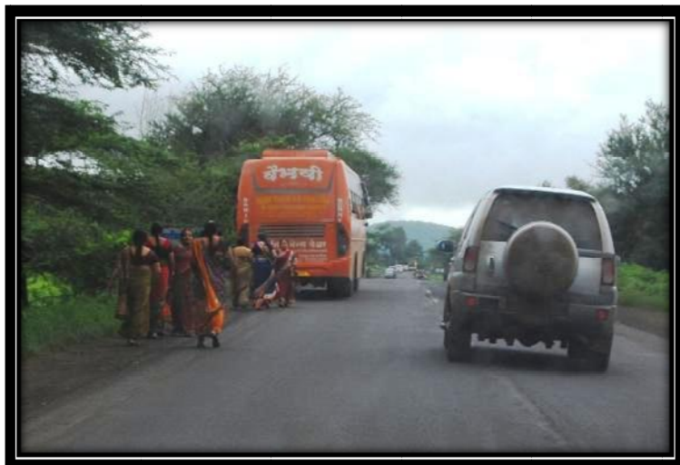
A bus stopped on a 1+1 lane undivided National Highway without much shoulder, creating safety hazards.
