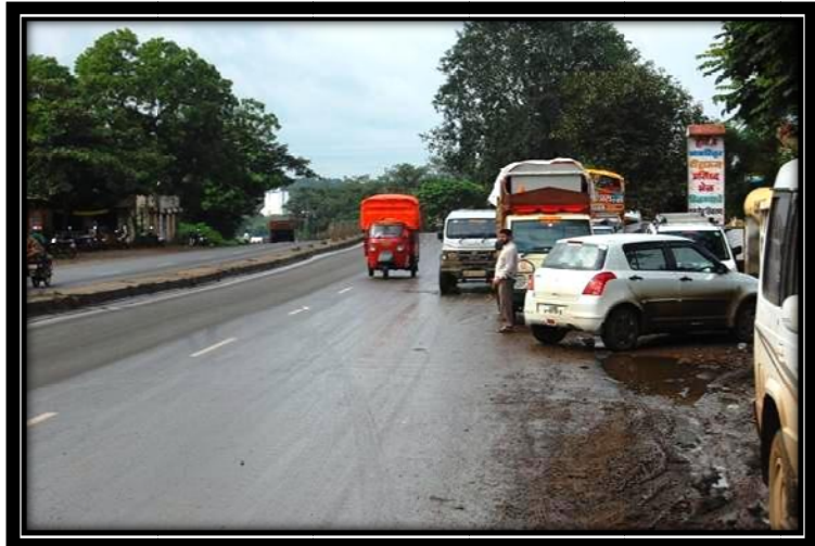
Vehicles do not have enough space to stop at the roadside and are stopped in the carriageway of this National Highway.
