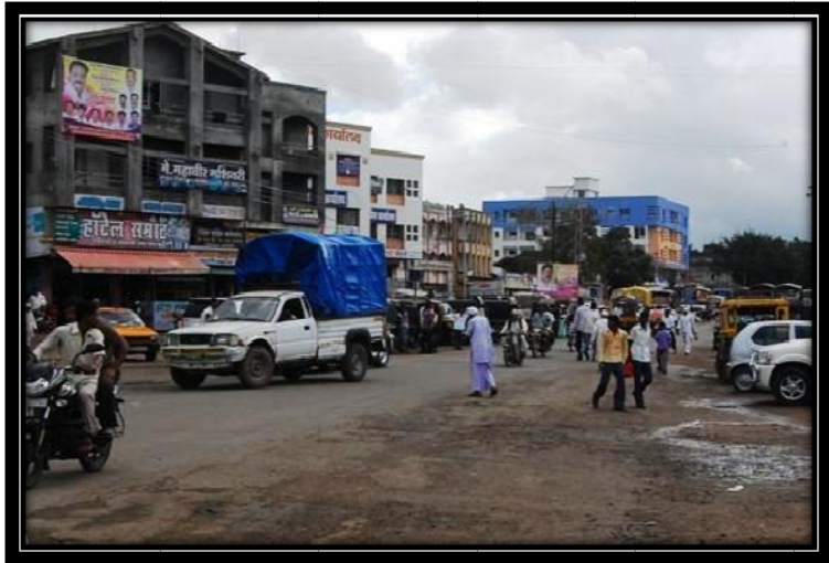
No road markings also means no designated safe place for pedestrians to cross.
