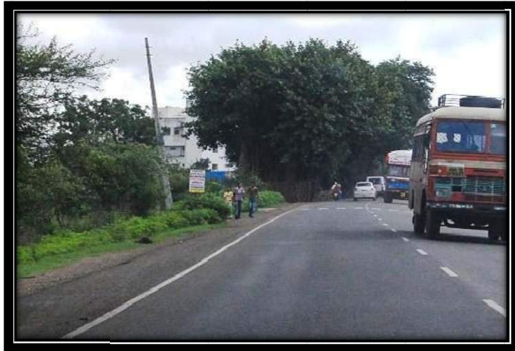
A clearly marked edge of the road and a proper shoulder makes walking along the NHs safer.
