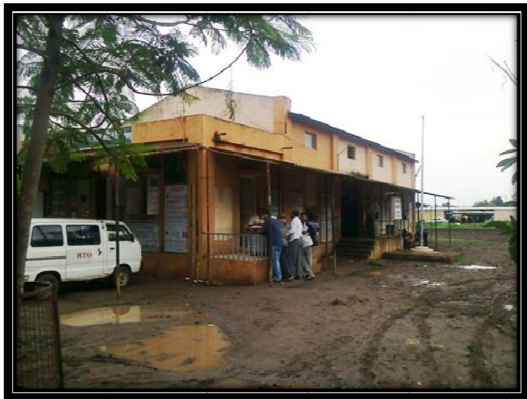
RTO building at Shrirampur, dist Ahmednagar.
